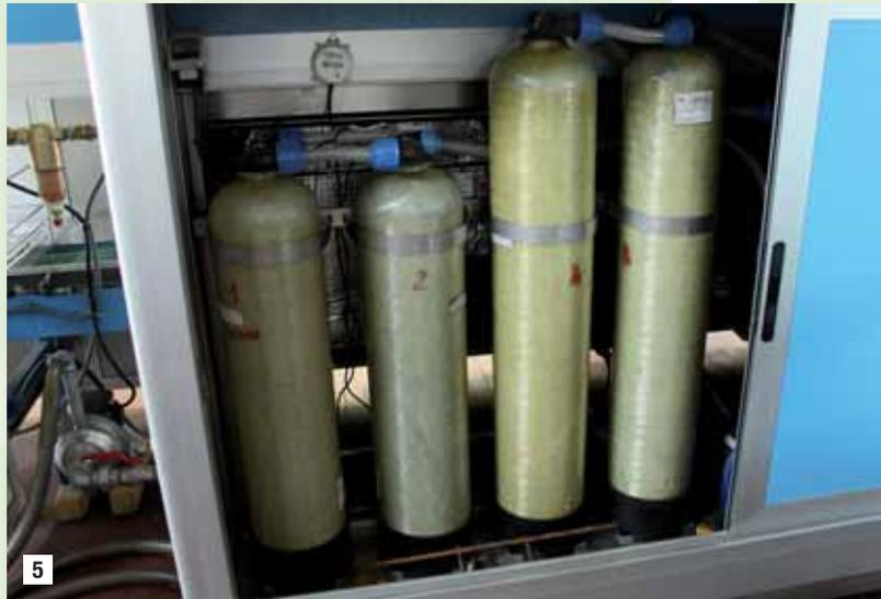
**5** *The cleaning system by MEG is equipped with columns of activated carbon and resins for the production of demineralised water needed for the final rinsing stage.*
