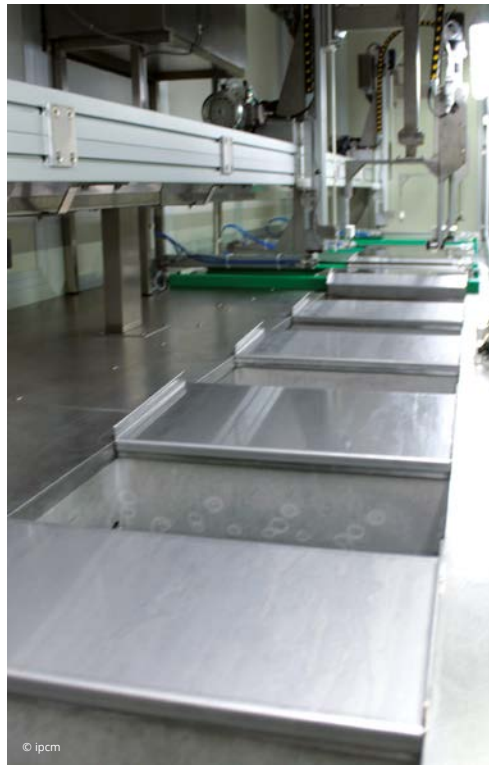
Some tanks in the plant.
