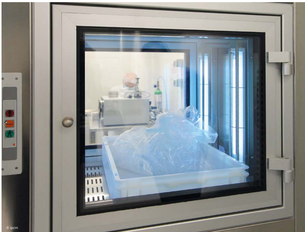
The pass box for transferring cleaned components to the clean room.
